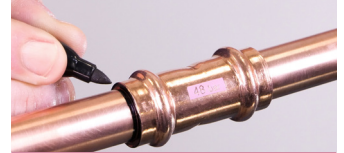
7B. Alternatively insert tube to tube stop and mark
