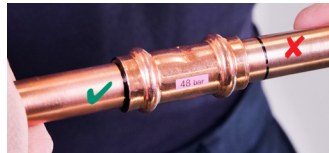
8. Insert the tube fully into the fitting. Ensure tube is fully inserted prior to pressing
