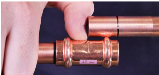
7B. Check the depth mark
